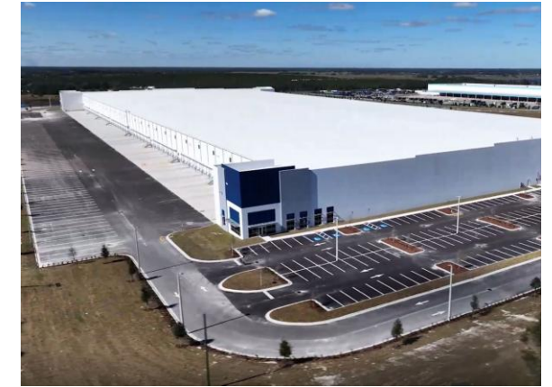
Apopka 429 – Building 400 NW Orange County Built: 23Q4 724,414 SF 0% leased
