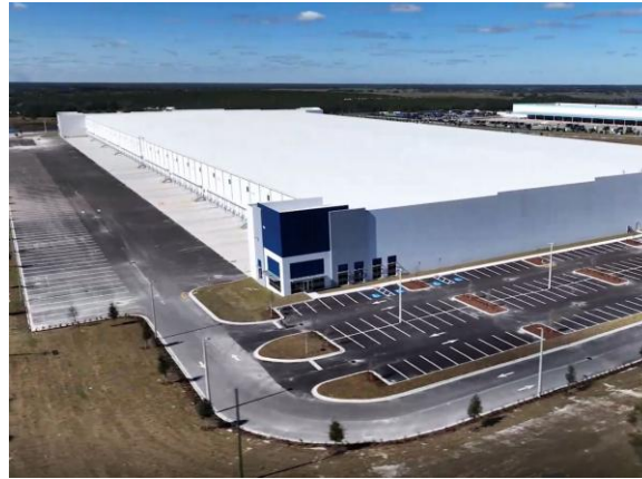
Turnpike Logistics Center Lake County Built: 23Q4 977,441 SF Leased to Duke Energy
